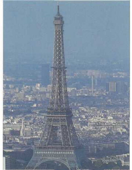
▼ Eiffel tower-Paris. Waterproofing of 2nd floor.
