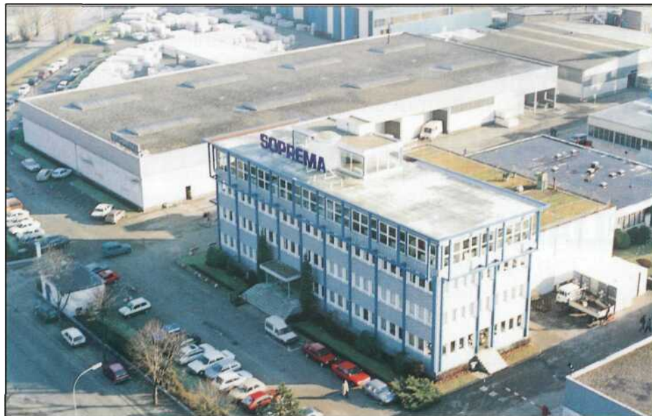
Plant and head-office in Strasbourg
