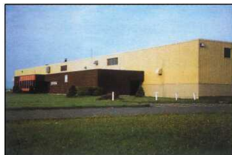
Plant in Drummondville - Canada
