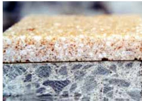
Sureshield topping on concrete slab
