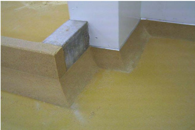
Nuthane Epoxy covers prior to Nuthane topcoat.
