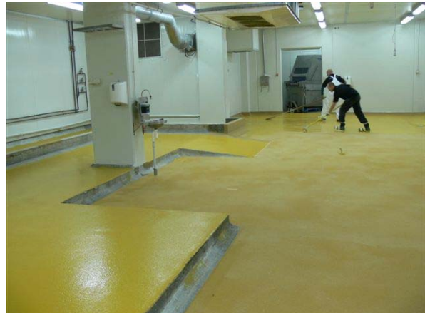
Application of Topcoat to Nuthane base.
